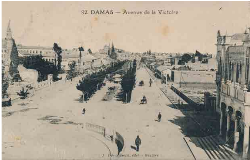
FIGURE 9.27 The square in front of the Hejaz Railway Station (to the right) and Cemal Pasha Boulevard (from a postcard in the collection of the author).
